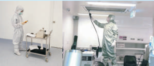
HVAC Validation of Pharma Industries
